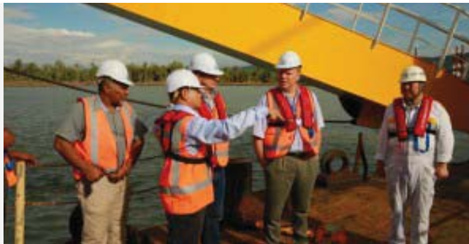
The ADB's Stephen Groff (2nd from right) inspects the Lae port development. (Credit: ADB).
