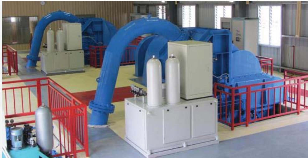
PNG Forest Products' power plant in Morobe Province. Credit: PNGFP
