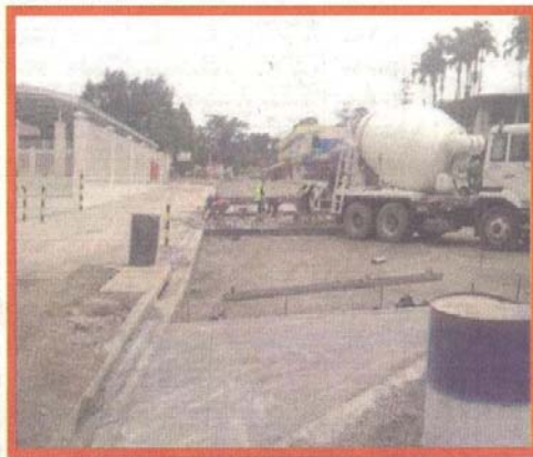
Pouring of Concrete Pavement in Progress
